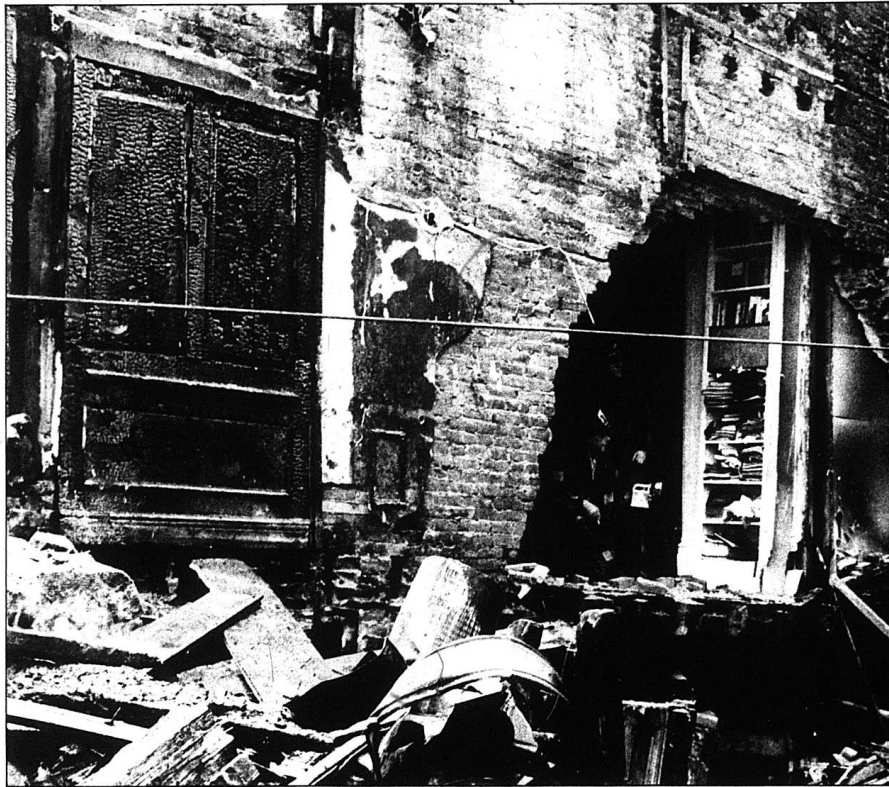
A gaping hole knocked out by a Fire Department crane ventilates Dustin Hoffman's second-floor apartment at Number 16.
